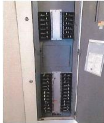
COURT BUILDING THREE (3) FEDERAL PACIFIC PANELS
